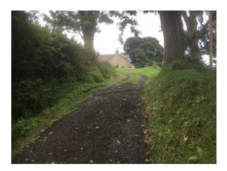
Although originally surfaced, the road has had no maintenance for many years leaing to the break-up of the surface and the encroachment and growth of vegetation. The width is less than that required for adoption in a rural setting and there are no passing places. The road is little better than a "dirt track".
