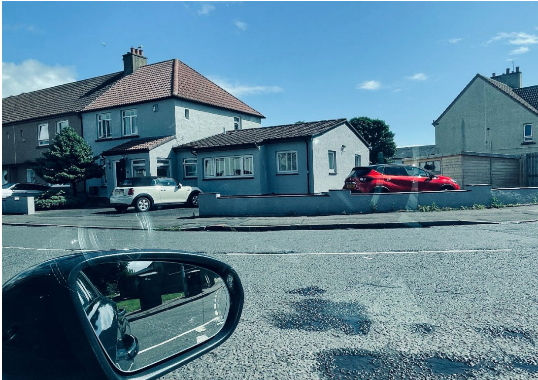
Photograph No3 – No13 Livingston Terrace, Irvine
