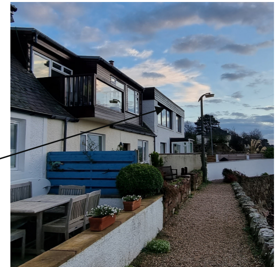
Existing end to the terrace with a flat roof
