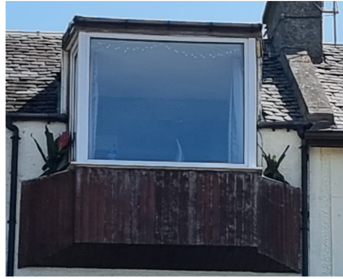
Vertical Timber Cladding
