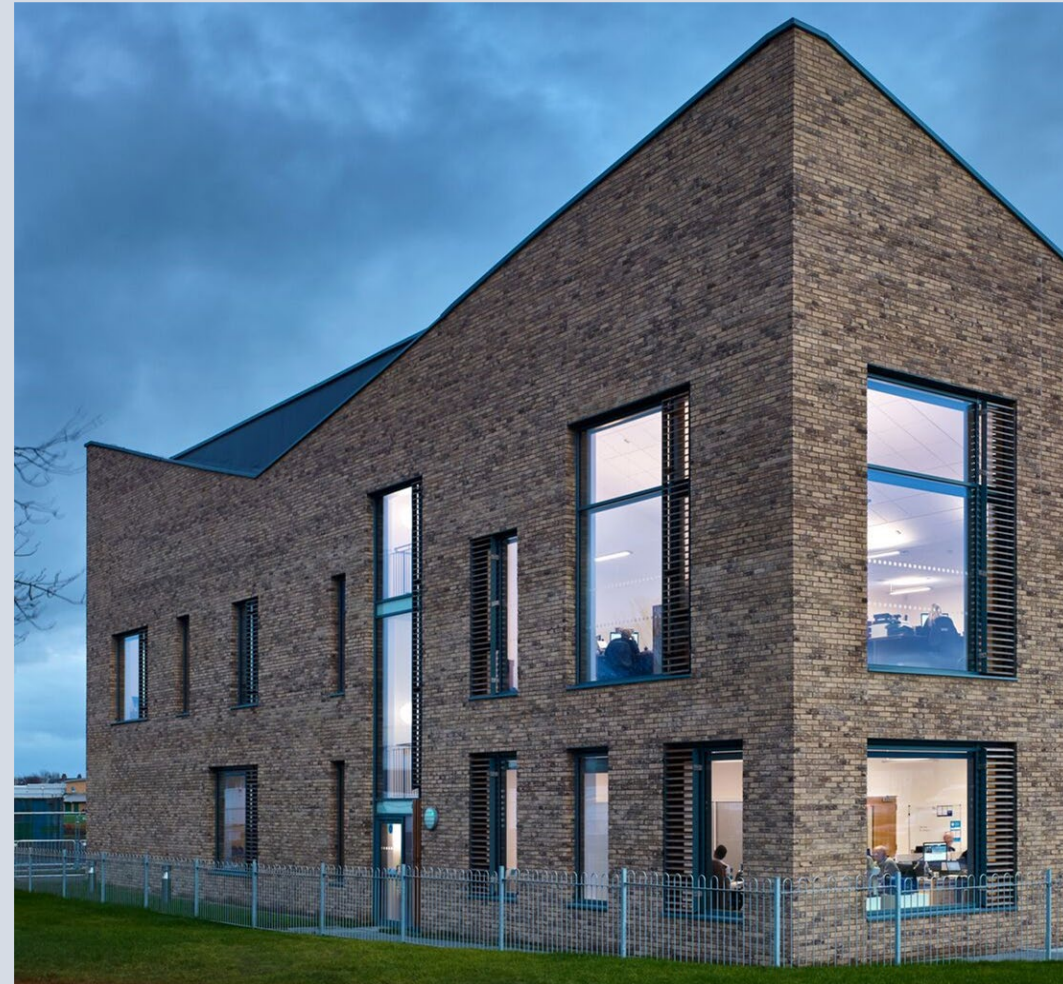
Redevelopment of derelict land at Quarry Road, Irvine.
