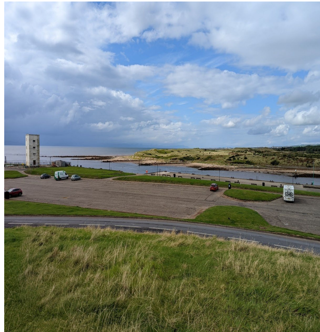
The pilot house at Irvine, within the proposed 'Maritime Mile' waterfront regeneration led by North Ayrshire Council.
