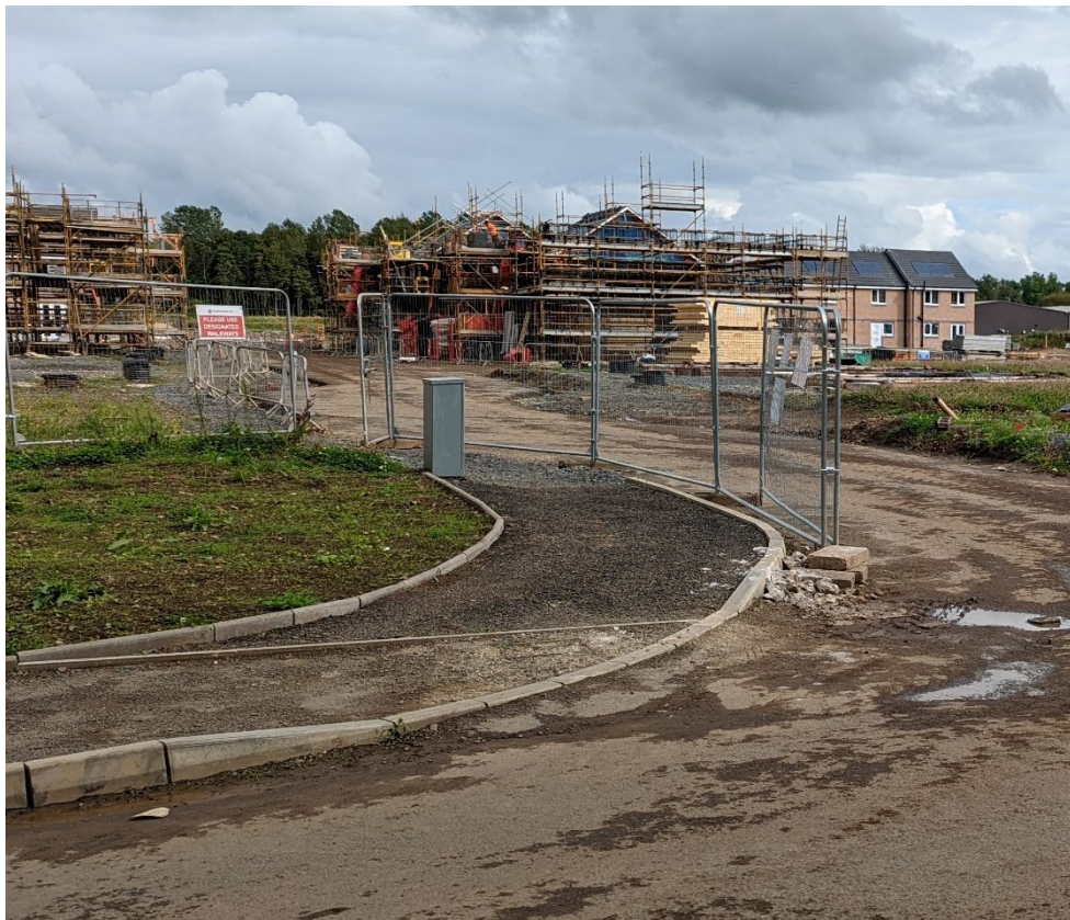
Housing on a previously derelict site at North Newmoor, Irvine
