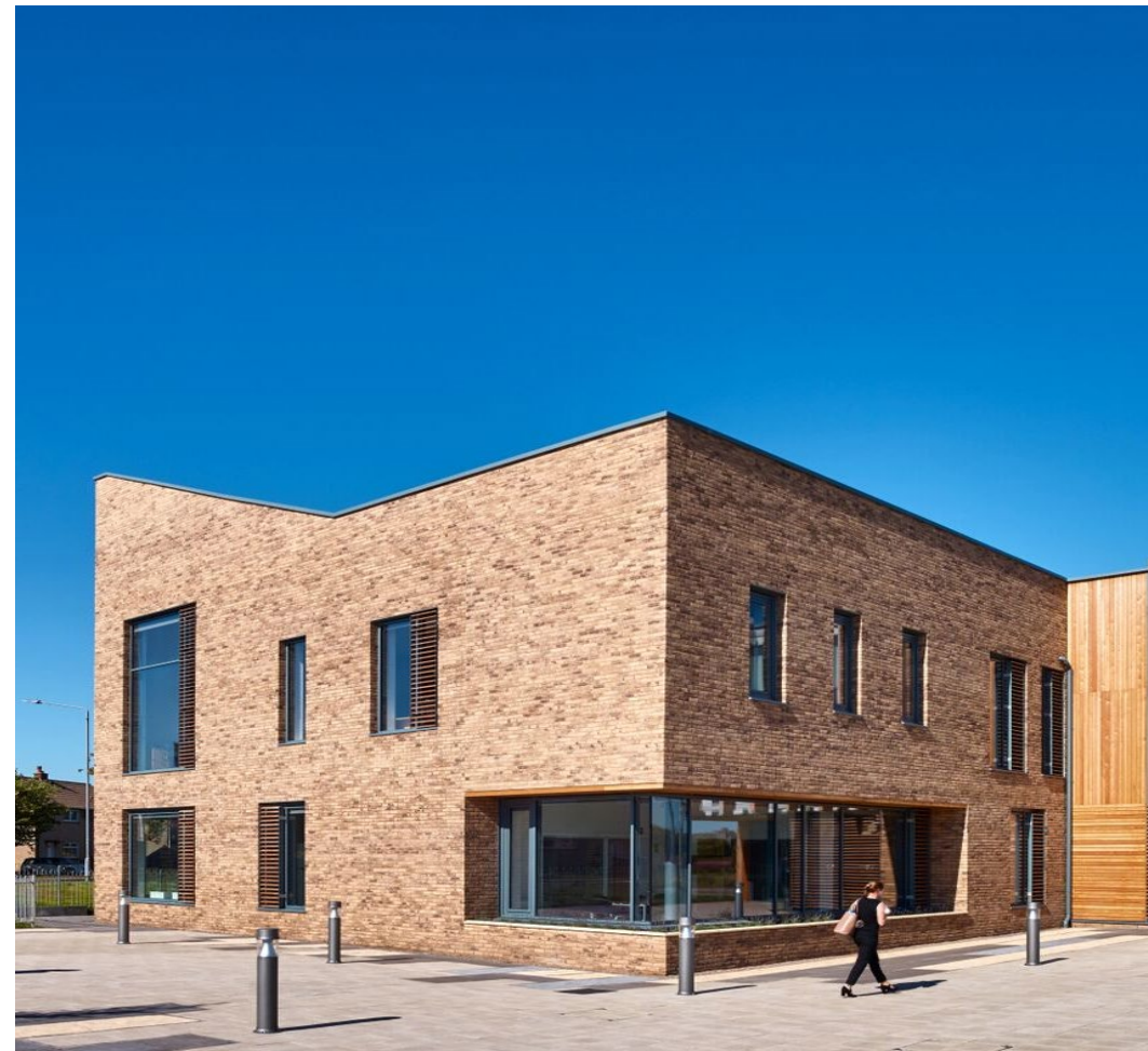
Quarry Road, Irvine.
