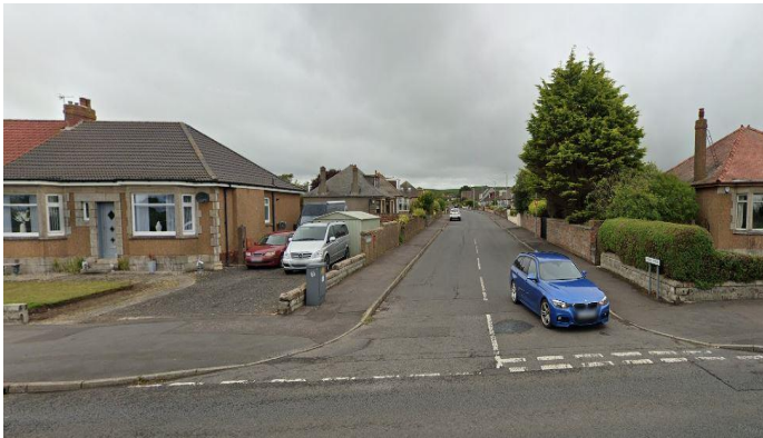
Photograph 1 - Junction of Murray Avenue and High Road, Saltcoats showing separation between adjacent houses
