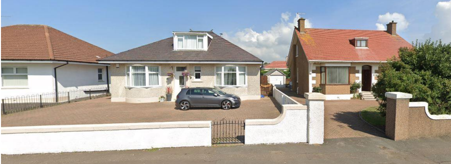
Photograph 3 - High Road, Saltcoats showing gabled roof adjacent to hipped roof
