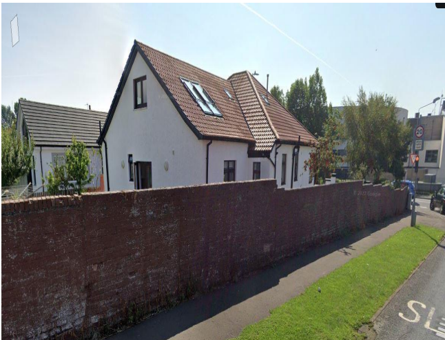
Photograph 2 - High Road, Saltcoats showing gabled roof extensions
