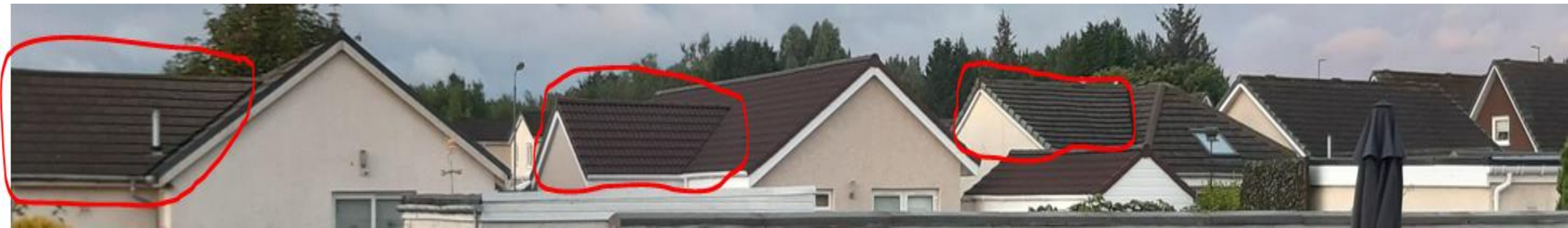
Examples of gable end style extensions on to side elevations of bungalows in Gray Crescent Irvine, within a few hundred metres of 8 Gray Crescent
