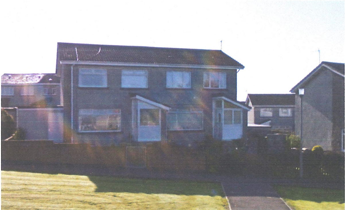
Picture 04 – Dalry Road, Saltcoats. These dwellings are facing West.
