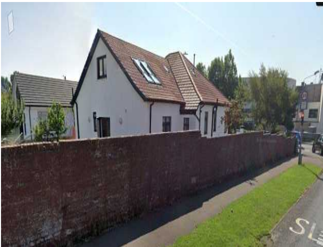
Photograph 2 - High Road, Saltcoats showing gabled roof extensions
