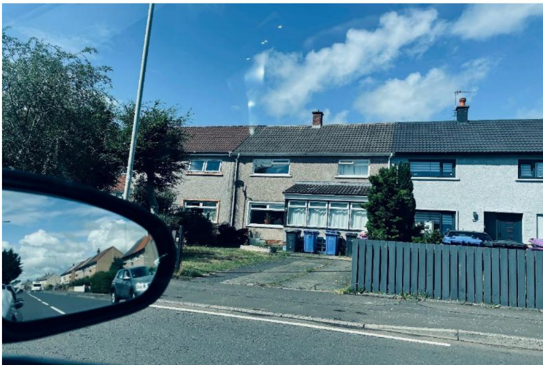
Photograph No4 – 68 Livingston Terrace, Irvine
