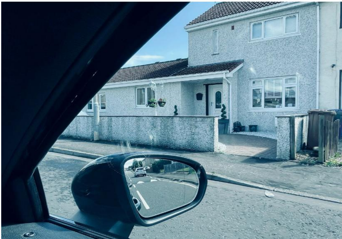
Photograph No2 – No179 Livingstone Terrace, Irvine
