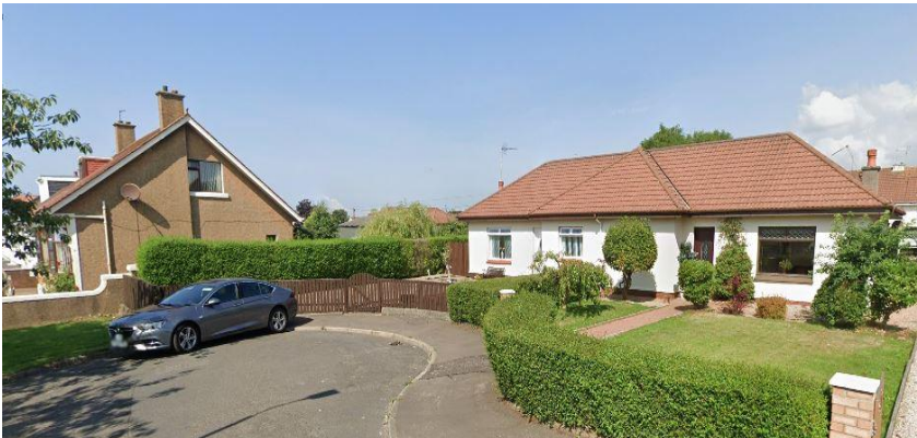
Photograph 4 - High Road, Saltcoats showing gabled roof adjacent to hipped roof
