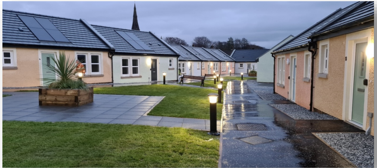
Supported accommodation at Bessie Dunlop Court, Dalry
