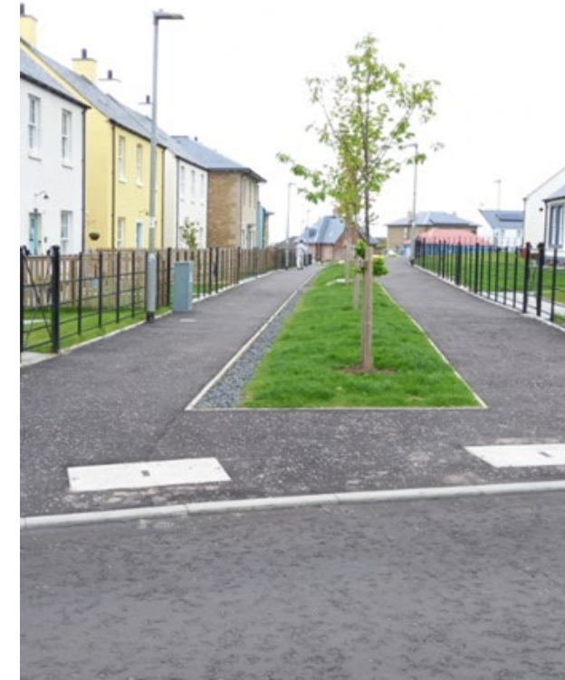
Figure 2 – Filter Trench for Rainwater Management
