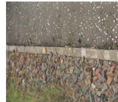
Figure 2 – Filter Drain
