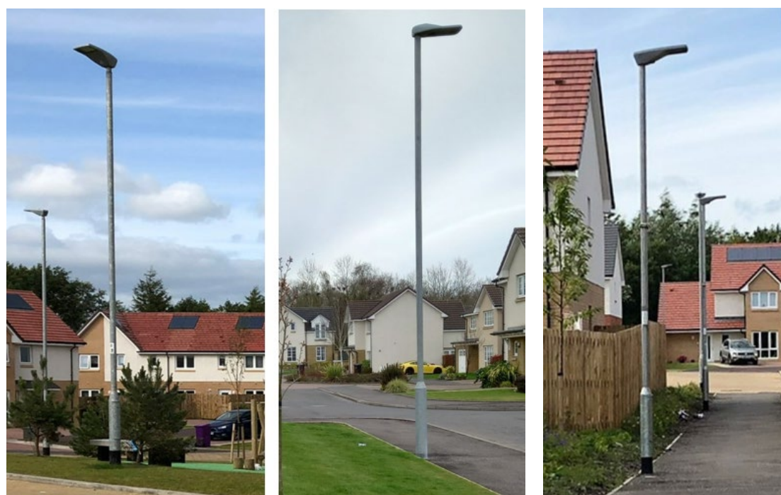
Figure 1 – Galvanised Finish Column Lighting with LED Lamps in Public Realm
