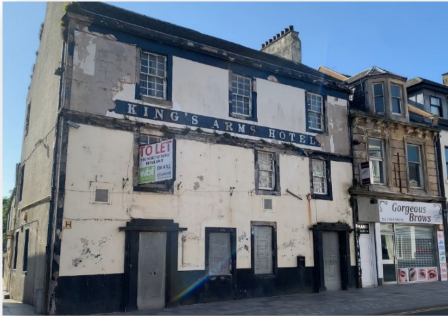
The Kings Arms located in Irvine Town Centre will be redeveloped to provide 6 new amenity flats
