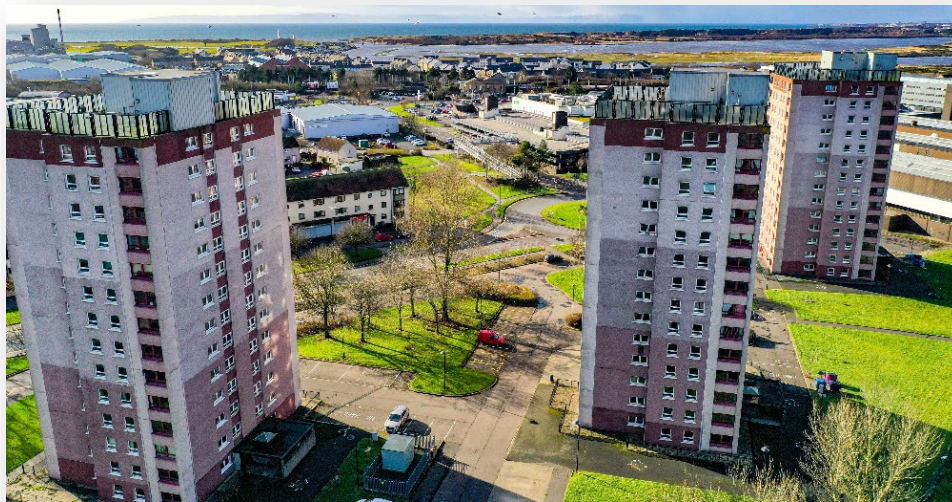
The Fullarton tower blocks in Irvine is a major regeneration project
