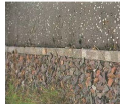
Figure 2 – Filter Drain
