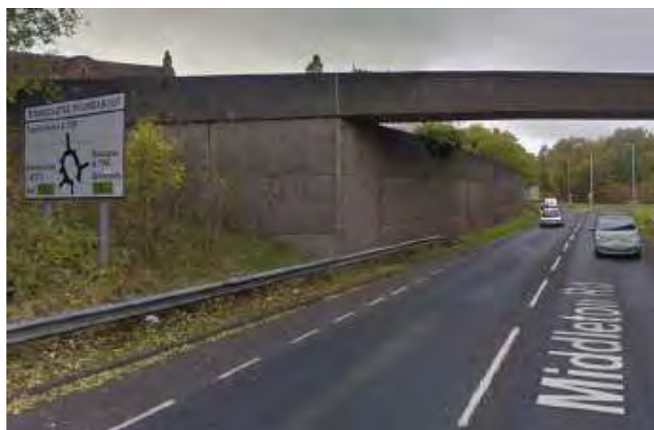
Figure 23. Retaining Wall and Crash Barrier Along Southern Verge of Middleton Road
