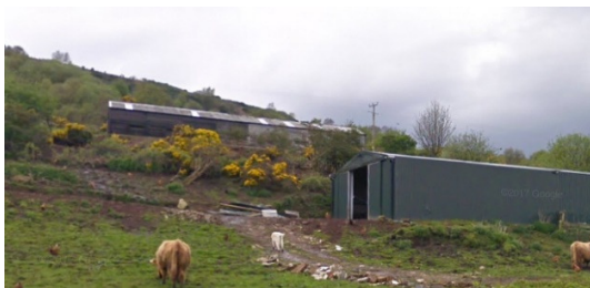
The current building from the road
