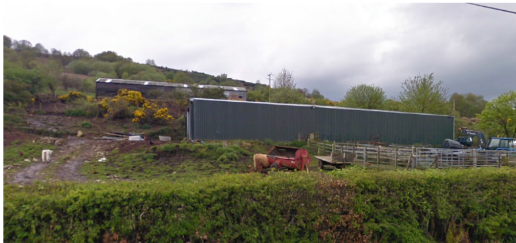
The former chicken shed sits in an elevated position above and behind a large agricultural shed to the West of the public road
