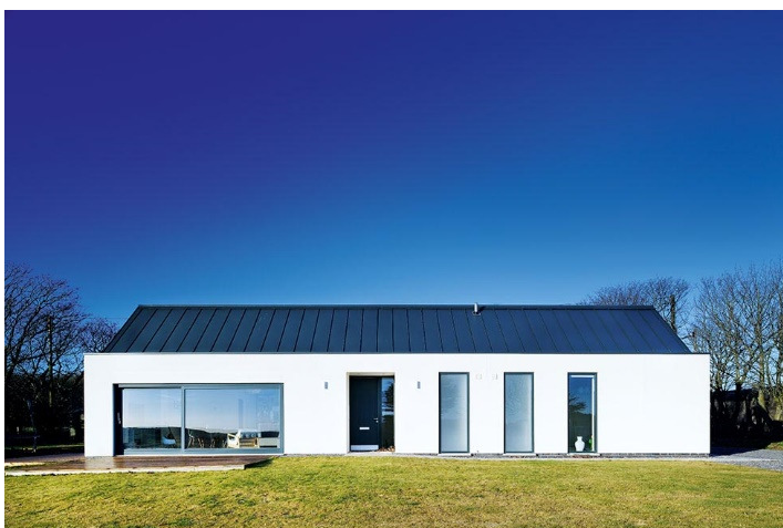
Private House, Aberdeen-shire
