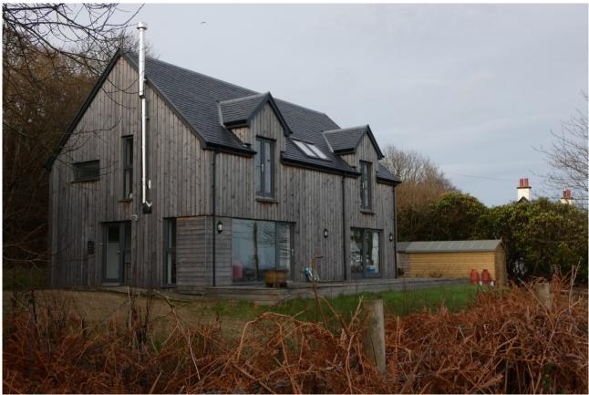
5. Larch Clad Building constructed in Whiting Bay showing weathered timber on the house and fresh timber on the adjacent garage
